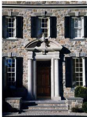
The limestone entry features iuscan columns topped with a broken pediment. Photo: Larry Landwehr
