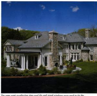
The same semi-weathering slate roof tile and wood windows were used to tie the structures together. Photo: Larry Landwehr
